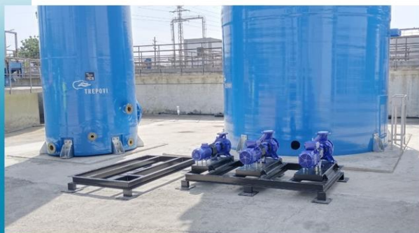
Pumps before mechanical assembly.
