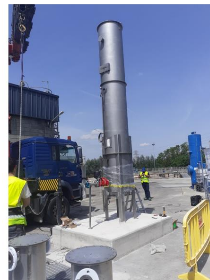
Flare being installed.
