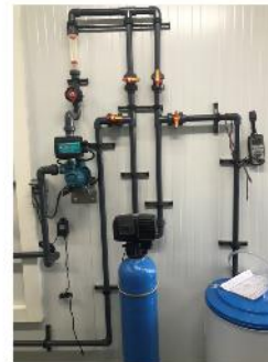
Adsorption with zeolites column
