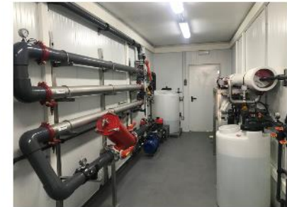
UF unit (left) and RO unit (right)
