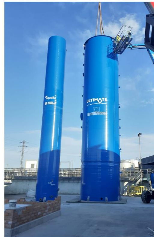
Buffer tank (left) and reactor (right). On the bottom left the retaining wall for emergency NaOH leakages can be seen
