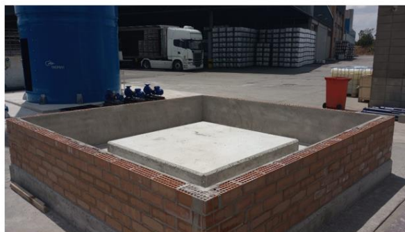
The retaining wall for emergency NaOH leakages.
