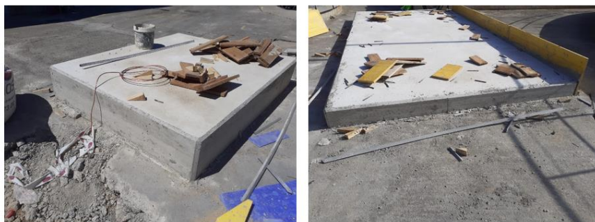
Concrete platforms for torch, gasometer and lamellar clarifier
